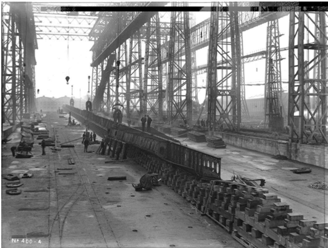
The layout of the keel is the first stage of the construction of a ship.
